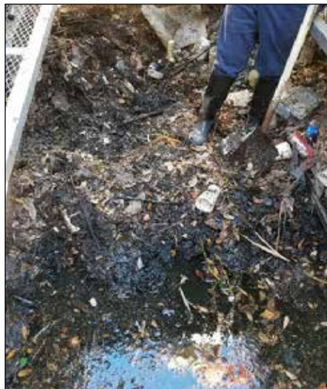
Figure 6. Pollutants collected by a nutrient-separating baffle box.
