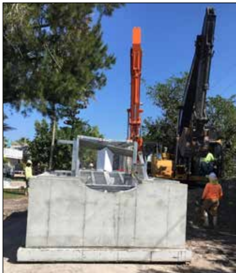
Figure 5. Lower half of nutrient-separating baffle box.
